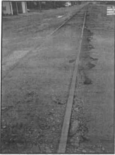
Example of a Rough Railroad Crossing
