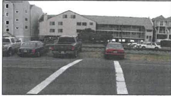
Lack of curb and gutter in southbound direction in downtown Rockaway Beach
