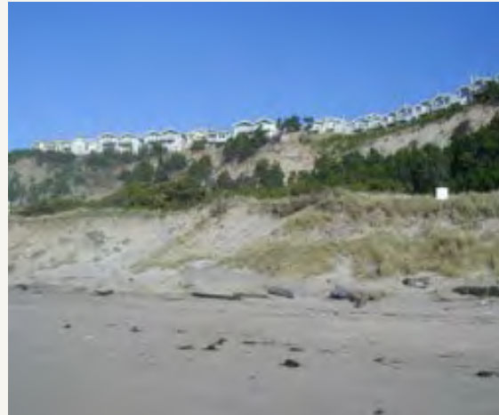
Figure 31. Erosion at “The Capes” Condominiums, Oceanside, Oregon
