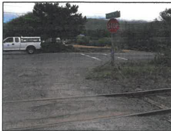
Washington St. railroad track crossing
