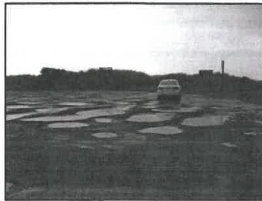
Existing Section Line Parking Lot
