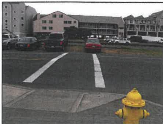
Lack of curb and gutter in southbound direction in downtown Rockaway Beach
