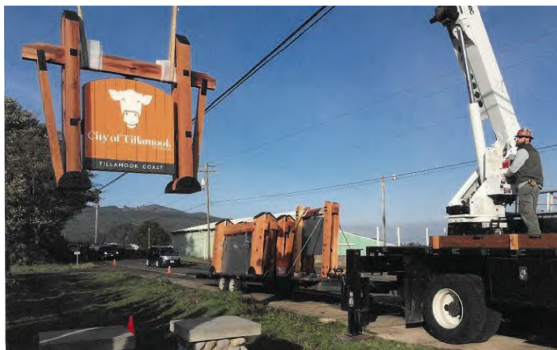
City of Tillamook Gateway sign installation
