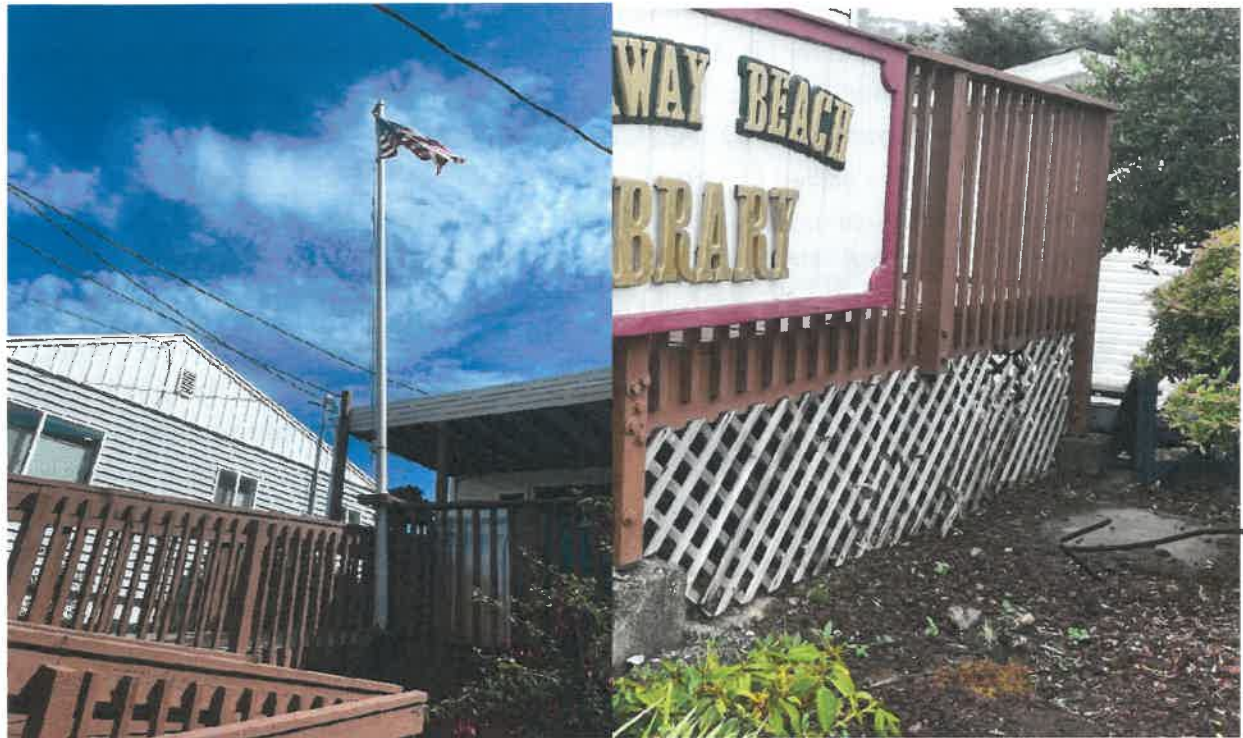
Where it is – just outside door on deck
