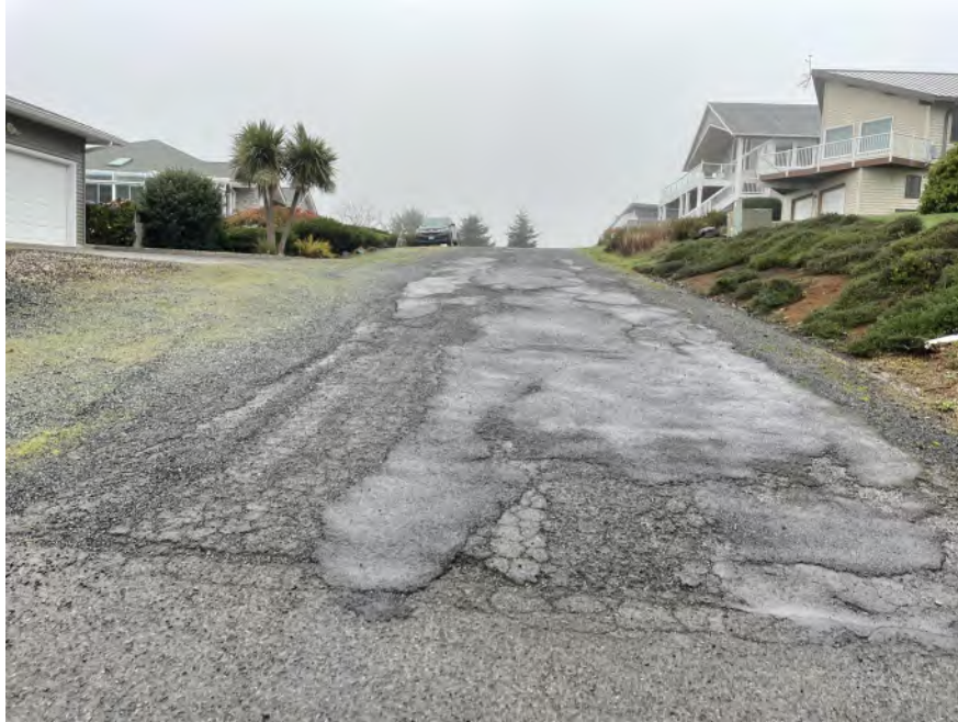
Figure 3-5 South Terrace Drive
