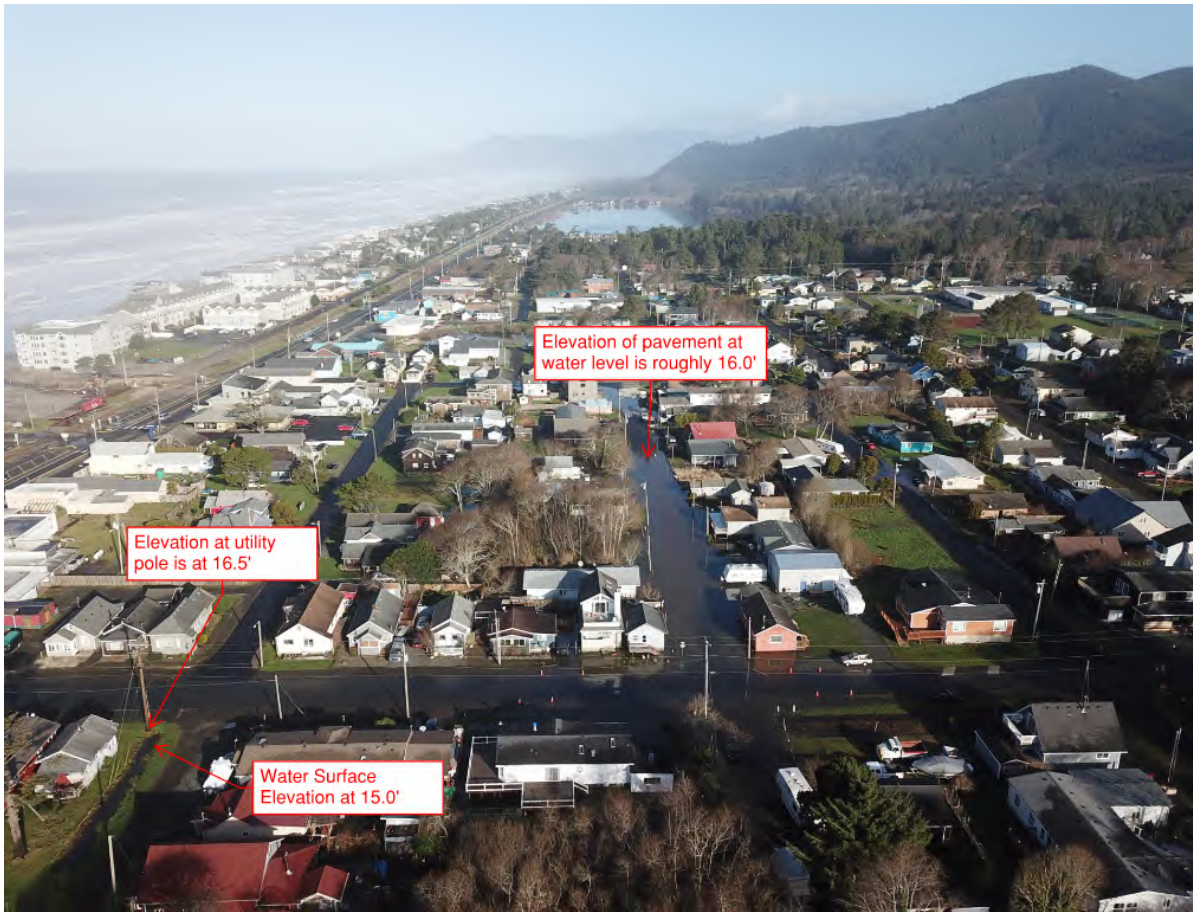
Figure 7 – Water Surface Elevation During Flooding
