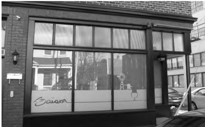
Sunshading and other screens may be necessary for your storefront, but should be removable like these blinds. Windows should not be permanently blocked, covered or reduced in size.
