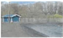
Wastewater Treatment Plant Willamina, OR
