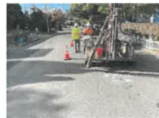
City of Oregon City, 2024 Pavement Maintenance Utility Fund Paving Project
