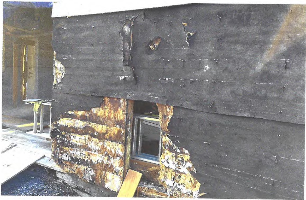
Plywood, Siding dry wall being replace the South side front half.
