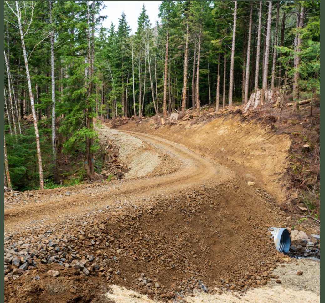
Photo: Road Construction – Arch Cape Forest
